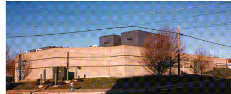
Network Access Point (NAP), operated by Sprint (in NJ)
