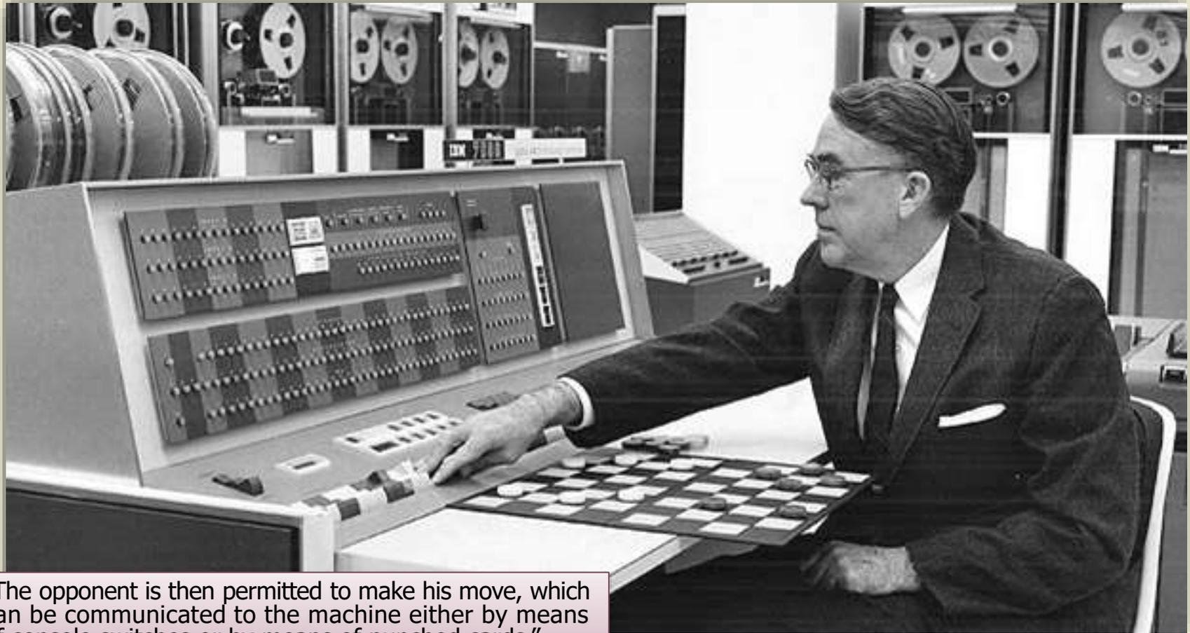
"The opponent is then permitted to make his move, which can be communicated to the machine either by means of console switches or by means of punched cards."
